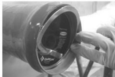
*Inserting Retaining Ring into the groove*
